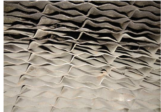
Fig 5: Double Undulated [DU] Profile
